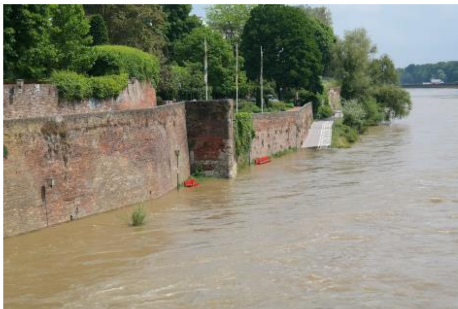
This image was taken in Ulm, Germany, when the river Danube (Europe's second longest river) caused flood damage due to excessive rainfall in June 2013. Hans/Pixabay
